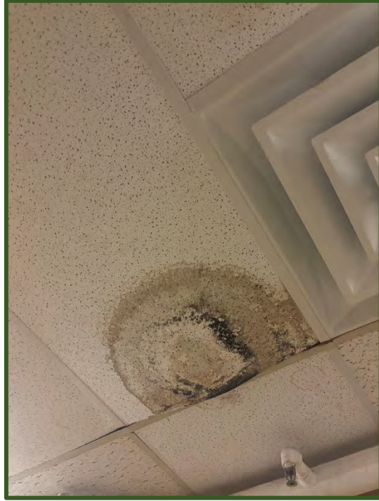
Figure 37 (left): Leak in ceiling in Dayton Hall.
