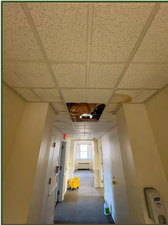
Figure 39 (left): Hole and stain from leak in ceiling of Erdman Hall.
