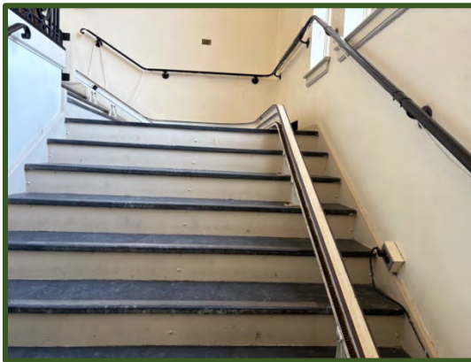
Figure 28 (left): Chair lift depicted in Bristol Hall, not accessible for wheelchair users. Figure 29 (right): Relocatable Classrooms, lacking in bathroom facilities.
