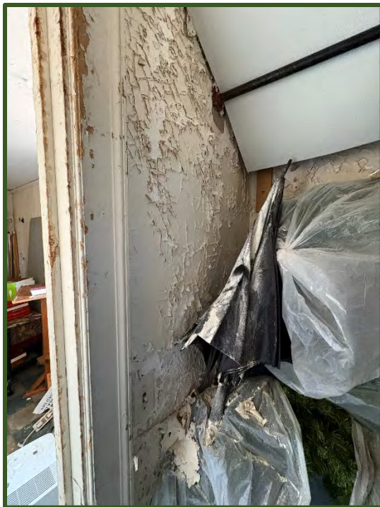
Figure 31 (left): Steam damage in Bristol Hall.
