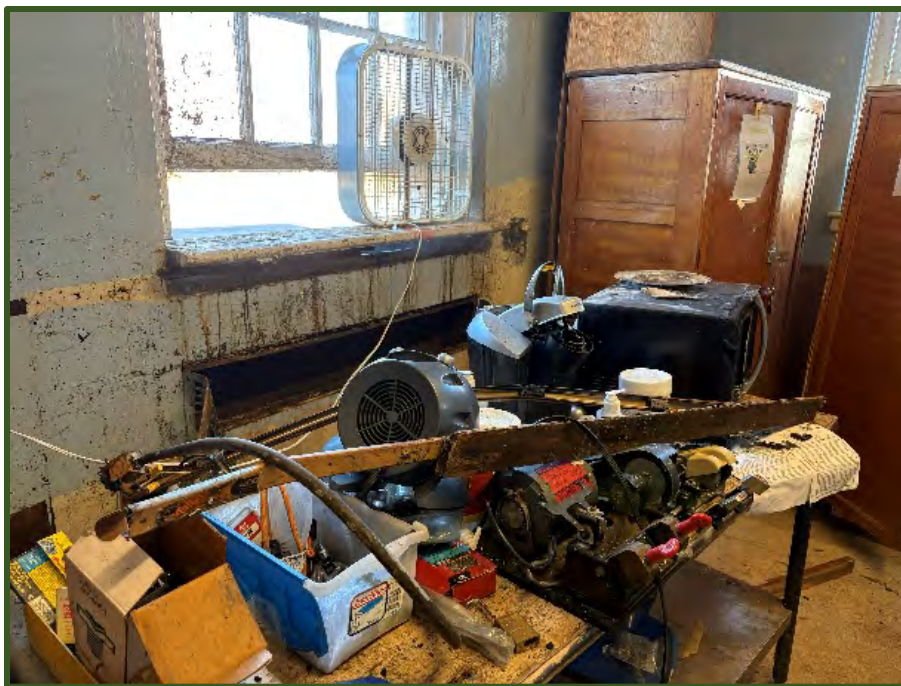
Figure 54: Evidence of fire related to the steam heating system that started on top of microwave in Bristol Hall.
