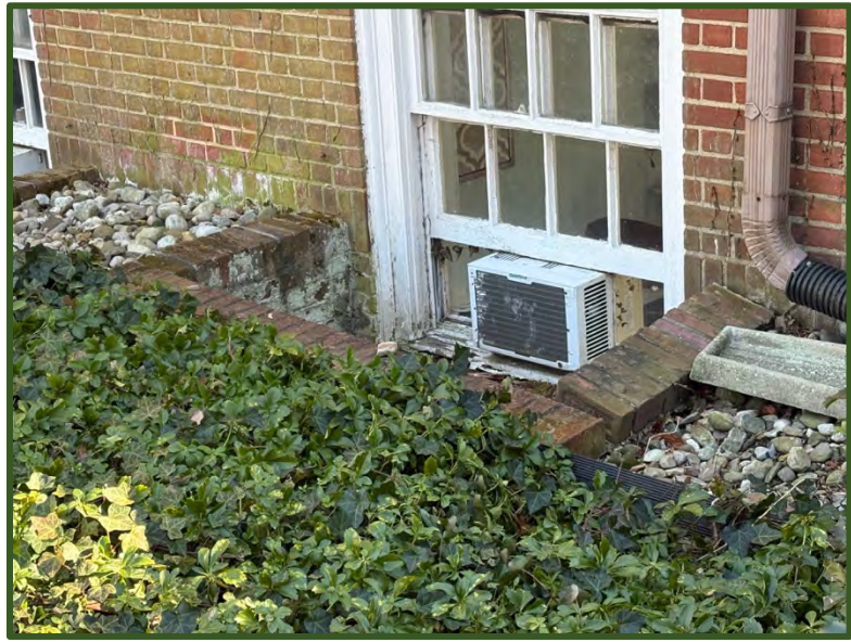
Figure 64: A window well in Williamson Hall depicted in dilapidated condition
