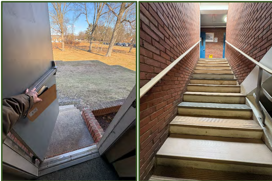
Figure 25 (left): Dorm exit, lacking accessibility features such as a hand railing.
