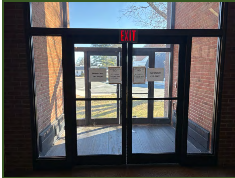
Figure 27: Exit/Entrance stairs which depict accessible exit with no sidewalk. Signs read "EMERGENCY EXIT ONLY!"
