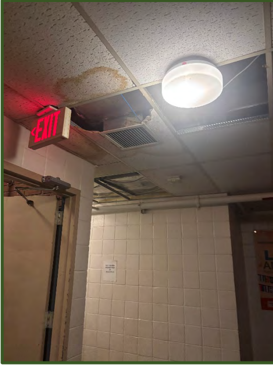
Figure 33 (left): Leak causing stain on ceiling in Princeton Hall. Figure 34 (right): Hole in ceiling depicting stain from leak in Ithaca Hall.
