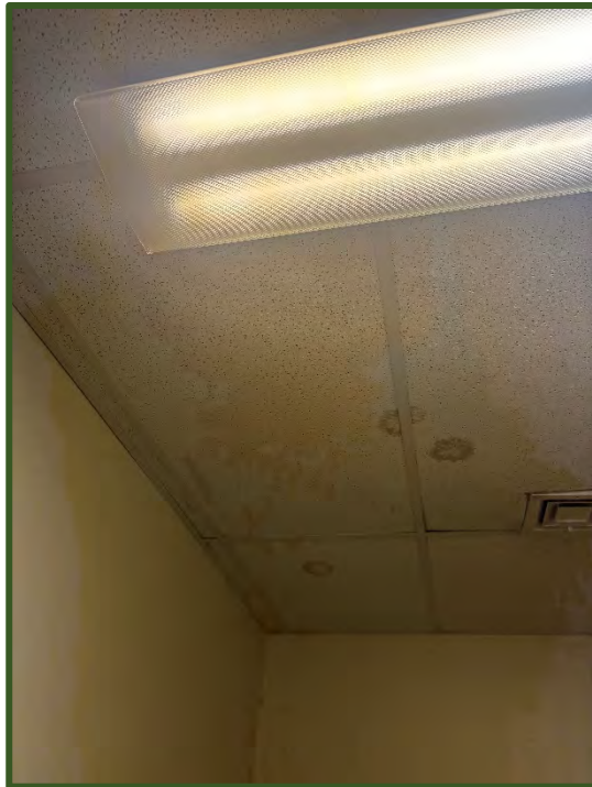
Figure 35 (left): Bucket on the floor of Ithaca Hall due to leak from ceiling. Figure 36 (right): Stains on ceiling of Ithaca Hall from a leak.
