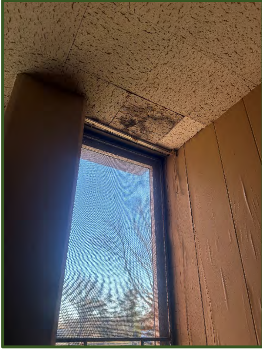
Figure 37 (left): Leak in ceiling in Dayton Hall.
