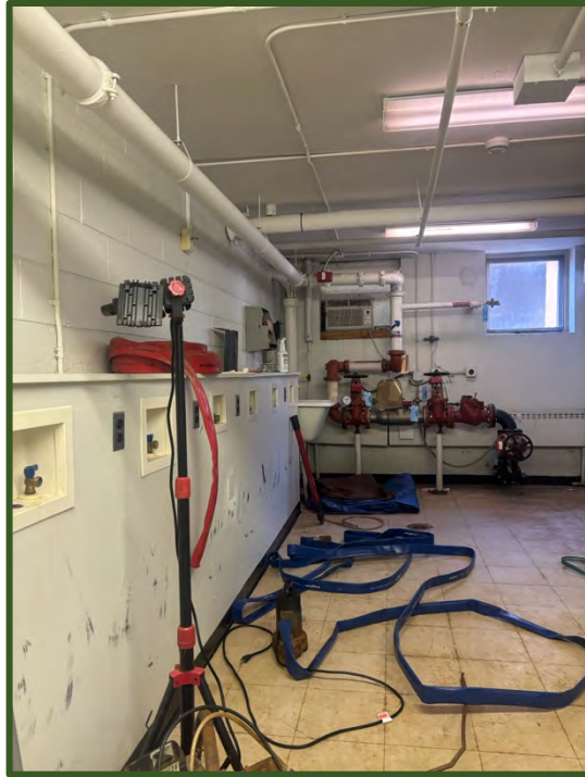
Figure 45 (left): Water damage alongside damaged plaster in Talbott Library
