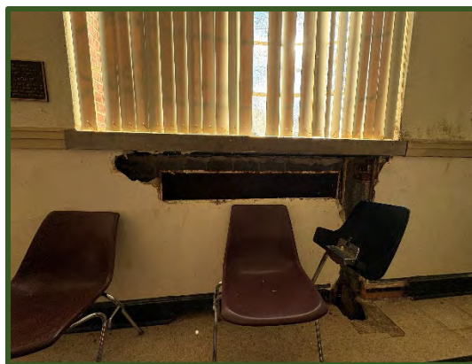
Figure 31 (left): Steam damage in Bristol Hall.
