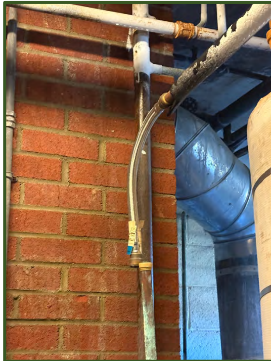
Figure 47 (left): Burst pipe that caused flooding in Seabrook Hall
