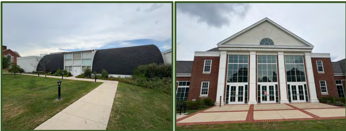
Figures 18-19: Robert L. Annis Playhouse (Left) and Cullen Center & Hillman Hall (Right)
