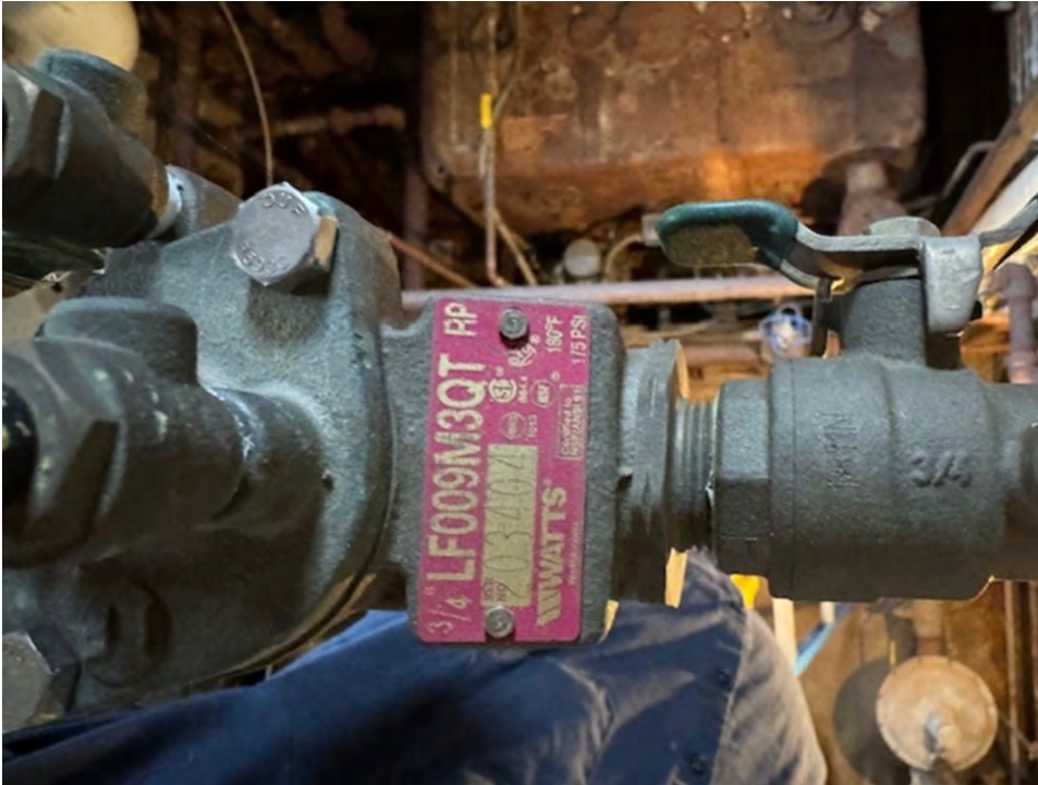
Backflow Preventer - Passed Certification
