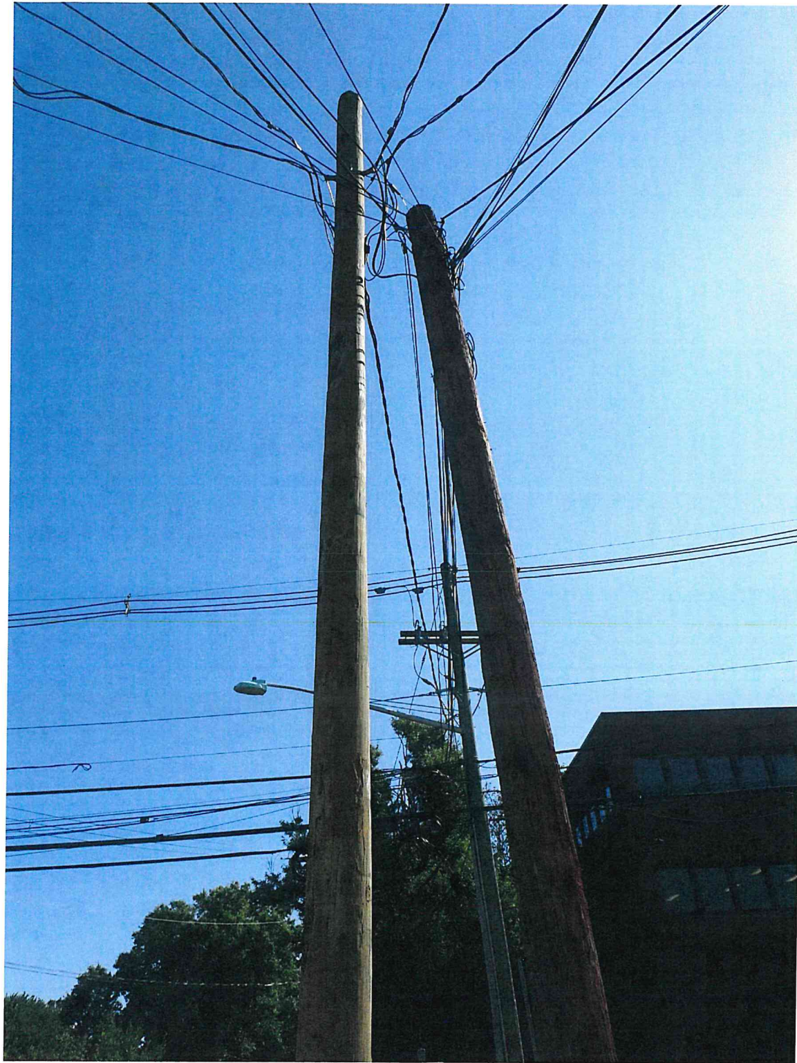
EXISTING POLE PHOTO LOOKING EAST
