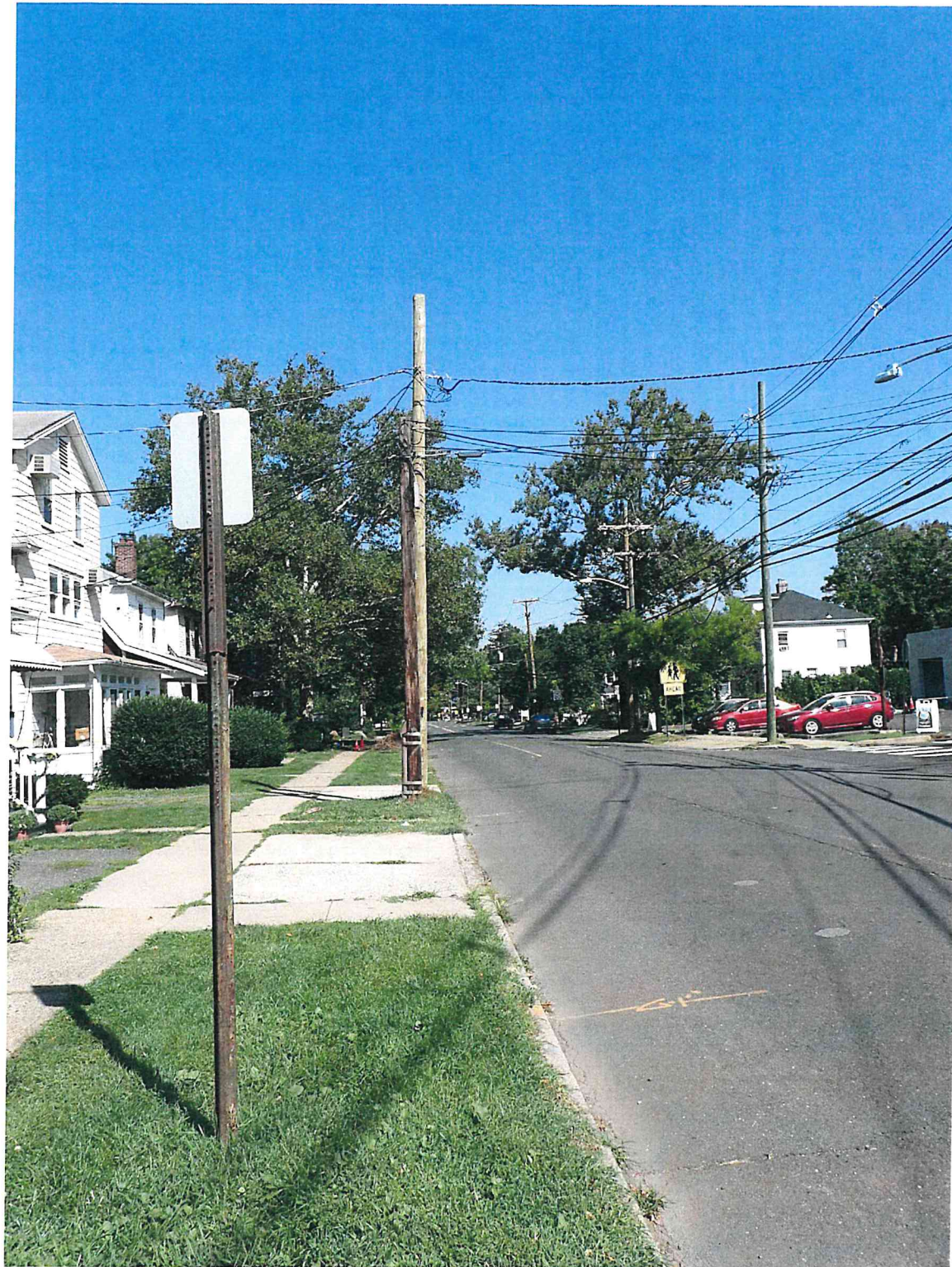
EXISTING POLE PHOTO LOOKING NORTH
