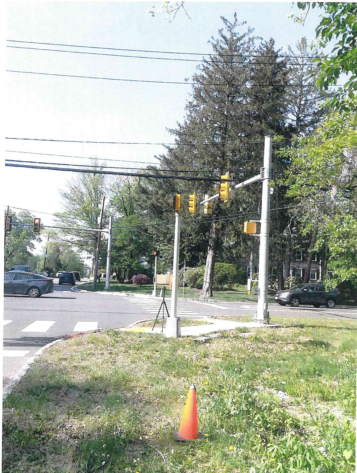
PROPOSED POLE LOCATION PHOTO LOOKING NORTH
