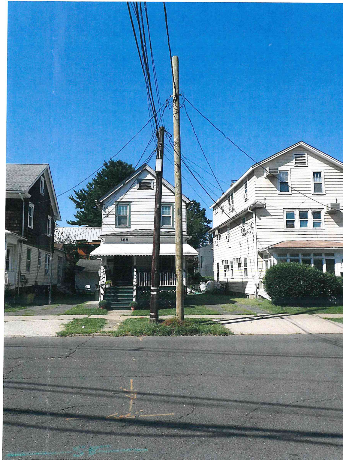
EXISTING POLE PHOTO LOOKING WEST
